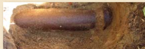
GLAZED TERRA COTTA WATER PIPES WERE DISCOVERED ON THE SOUTH SIDE OF THE PRINCIPAL KEEPER'S DWELLING.
