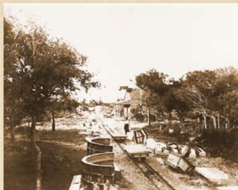
A TRAMWAY WITH A MULE-DRAWN CART WAS USED TO MOVE SUPPLIES FROM THE RIVER LANDING TO THE TOWER CONSTRUCTION SITE.
