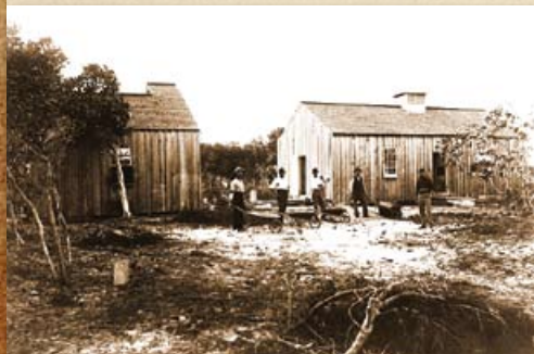
TEMPORARY KITCHEN AND QUARTERS WERE BUILT FOR THE MEN WHO CONSTRUCTED THE LIGHT STATION.
