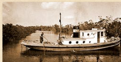
BOATS SUCH AS THE ONE ABOVE WERE USED DURING THE BUILDING OF THE INTRACOASTAL WATERWAY.
