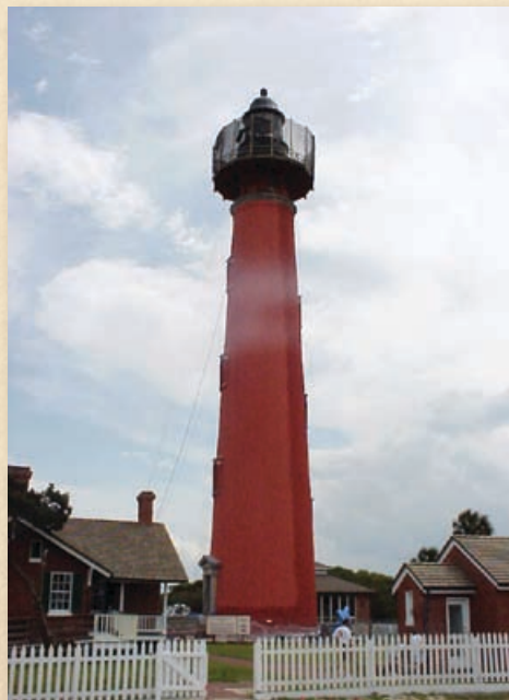
THE TOWER UNDERGOES COMPLETE RESTORATION IN 2000
