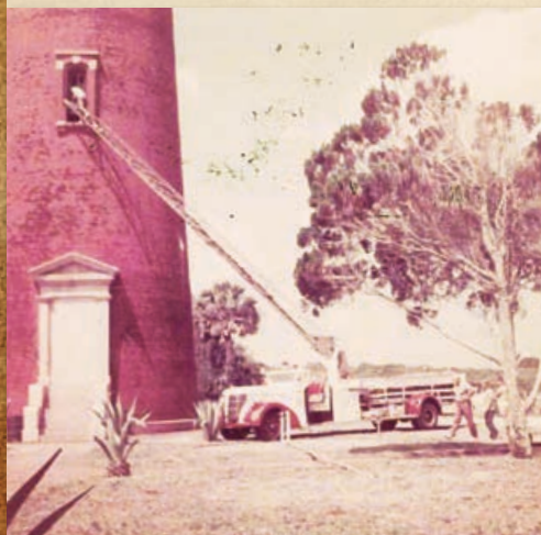
IN EARLY 1972, THIS WAS THE ONLY WAY TO ENTER THE TOWER.
