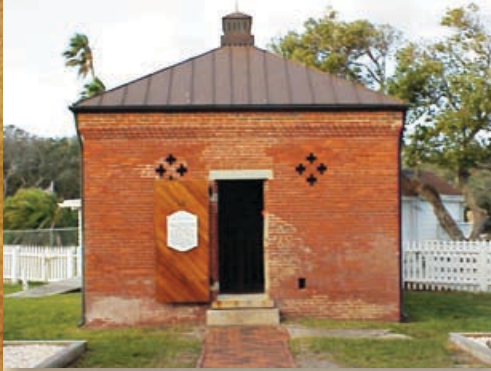
THE RESTORED OIL HOUSE
