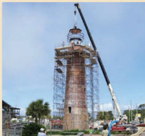
THE TOWER GETS ITS LANTERN ROOM
