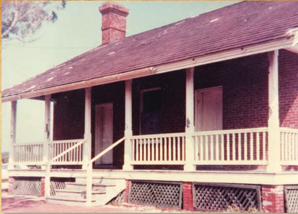
THE SECOND ASSISTANT KEEPER'S DWELLING BEFORE RESTORATION
