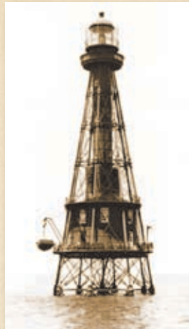
CAST BY THE PHILADELPHIA BASED I.P. MORRIS COMPANY IN 1858, THE SHIP SHOAL LIGHTHOUSE IS A CAST IRON SCREW PILE LIGHTHOUSE LOCATED OFF THE COAST OF LOUISIANA
