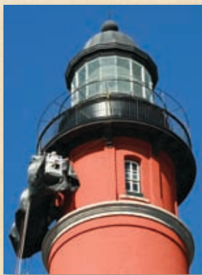
H.I.S. EMPLOYEES PAINT THE FINAL DECK SECTION
