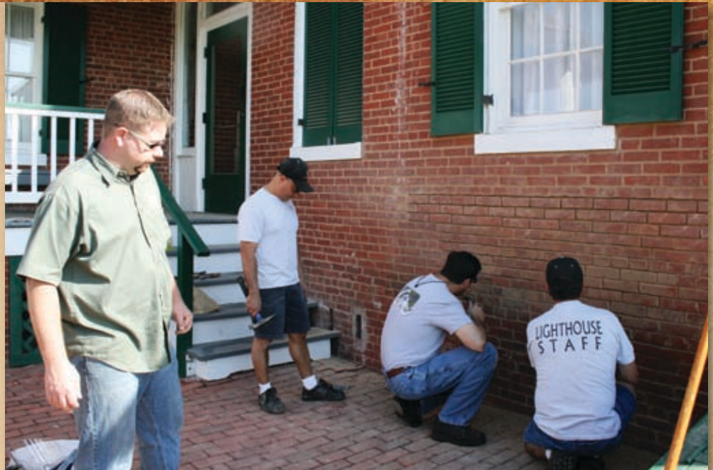
AARON WOLK OVERSEES REPOINTING ON BUILDING 5
