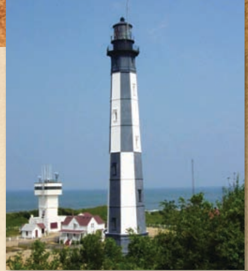
STANDING 163 FEET TALL, THE CAPE HENRY LIGHTHOUSE IS THE TALLEST CAST IRON LIGHTHOUSE IN THE UNITED STATES
