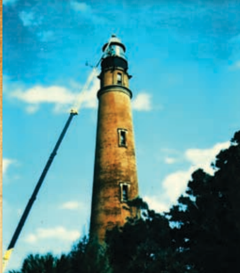
THE TOWER RECEIVES A NEW GALLERY DECK IN 1982
