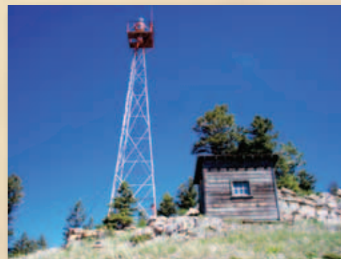
WOLF CREEK BEACON AND NEARBY SHELTER FOR MAINTENANCE WORKERS. COURTESY OF MIKE ROGAN
