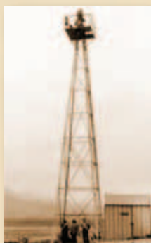
TYPICAL 51 FOOT TOWER WITH ROTATING SEARCHLIGHT
