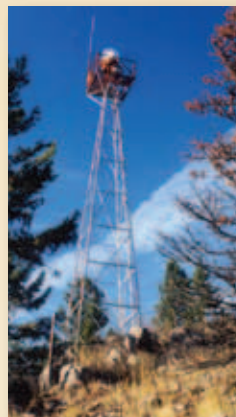
MONTANA LIGHTED AIRWAY BEACON TOWER. COURTESY OF MIKE ROGAN
