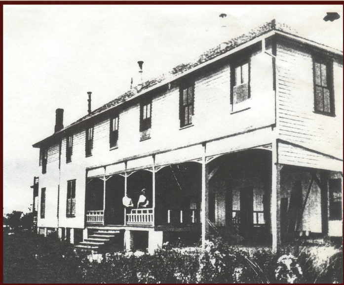
The Pacetti Hotel once had a large rear porch.
