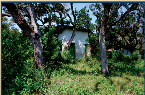
The property includes several outbuildings in need of repair
