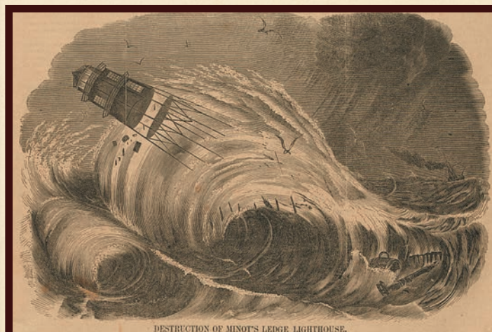
The original iron-pile Minot's Ledge Lighthouse collapsed into the sea during a violent storm outside Boston Harbor in 1850.
