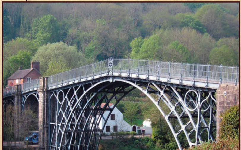
The 17th Century Cast Iron Bridge still stands today.
