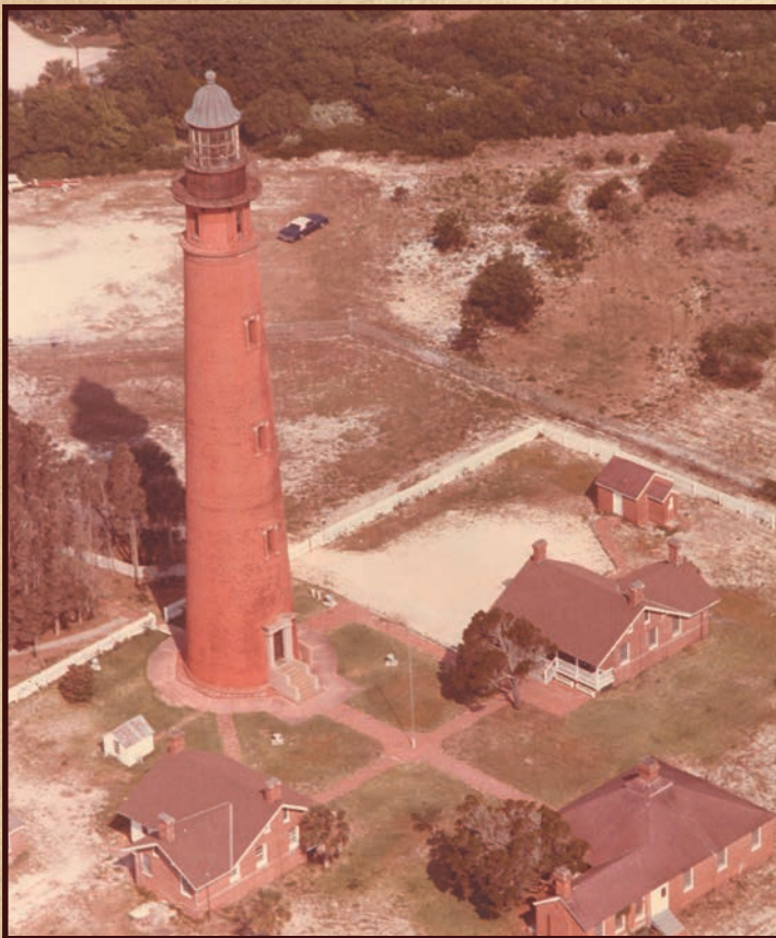
Although once meticulously maintained, twenty years of neglect had caused the lighthouse to fall into a state of disrepair.
