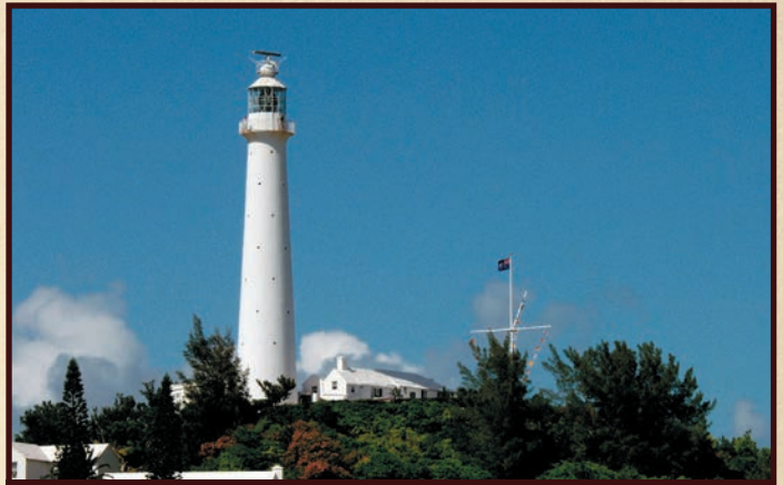
Erected in 1844, the cast iron Gibbs Hill Lighthouse was fabricated in England and then exported to Bermuda.
