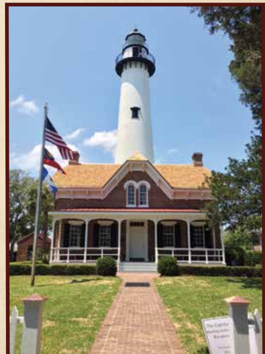
The St. Simons Lighthouse and the restored keeper's dwelling
