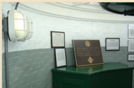
THE INTERIOR OF THE TOWER AFTER RESTORATION
