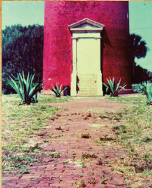
AN OVERGROWN BRICK WALKWAY LEADS TO THE SEALED TOWER ENTRANCE IN 1972.
