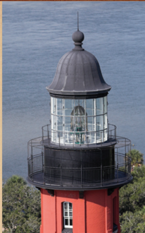
IN 2004, THE PRESERVATION ASSOCIATION RETURNED THE NEWLY RESTORED 3RD ORDER LENS TO ITS ORIGINAL HOME AT THE TOP OF THE LIGHTHOUSE.
