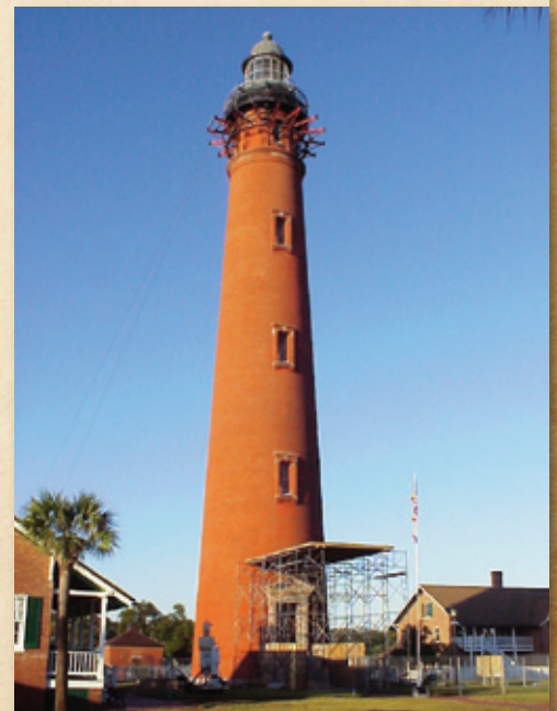
THE TOWER UNDERWENT A COMPLETE RESTORATION IN 2001
