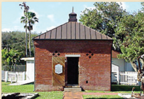
THE OIL STORAGE HOUSE WAS RESTORED BY THE ASSOCIATION IN 1989.
