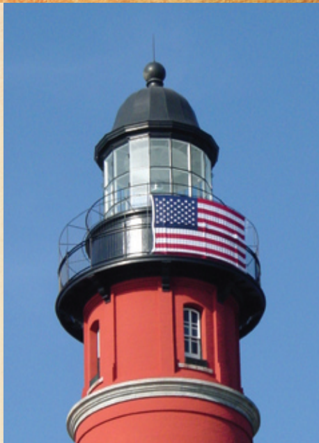
THE TOWER'S EXTERIOR METALWORK WAS RESTORED BETWEEN 2010 & 2011
