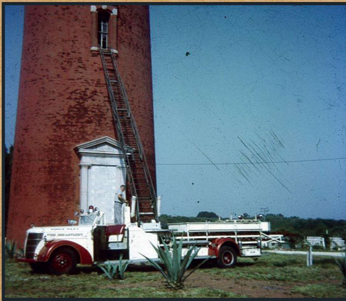
The Coast Guard sealed the entrance of the tower with concrete block in 1970 to prevent trespassers from entering the lighthouse. The Ponce De Leon Inlet Lighthouse Preservation Association initially used an old fire truck to enter the tower through the first window to begin their restoration and preservation efforts in the early 1970s.
