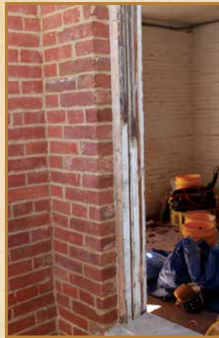
Masonry restoration around the Generator Room's east facing window is complete.
