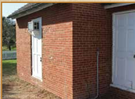
The entire south wall of the Generator Building has been repointed.
