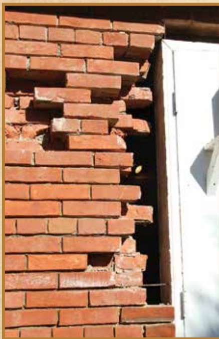
The area around the south door required substantial work.
