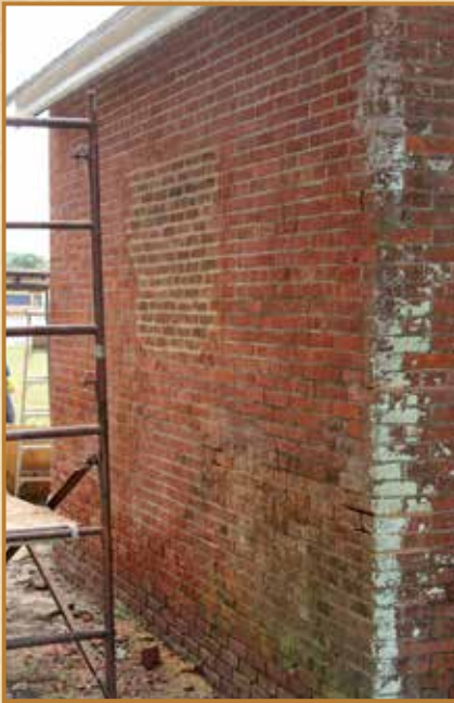
The completed restoration of the principal keeper woodshed's east wall.
