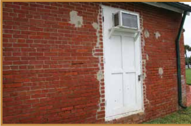
South wall of the Generator Building before repair.
