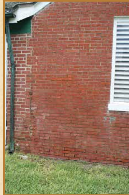
The joint between modern and historic sections of the Generator Building.
