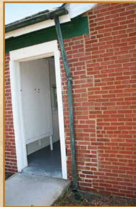
The completed repair on the Generator Building's west side.
