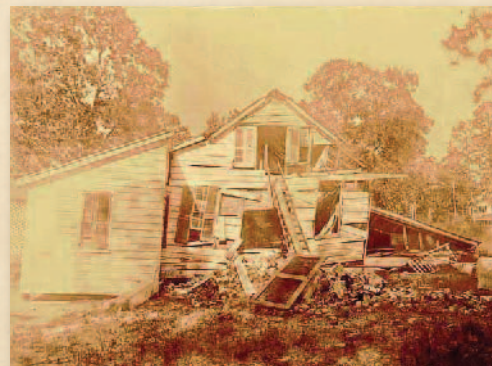
HOUSE IN SUMMERVILLE
