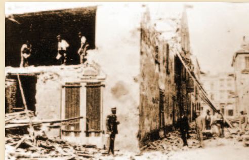
DAMAGED WAREHOUSE IN CHARLESTON
