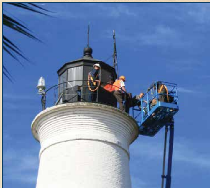
The lens is positioned in the man lift basket.
