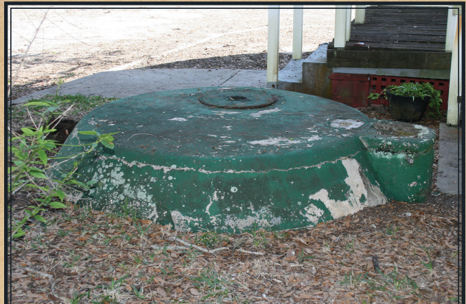
Cistern #2, constructed around the same time as the hotel addition, has a more sophisticated design than cistern #1; collection of the Ponce De Leon Inlet Lighthouse Preservation Association.
