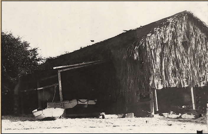
The original thatched boat house at the Mosquito Inlet Light Station; collection of the Ponce de Leon Inlet Lighthouse Preservation Association
